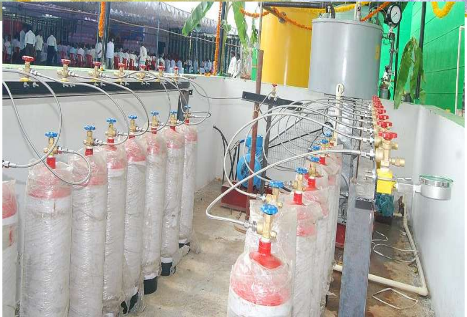
Compressed biogas cylinders at Maltose Agri Products Pvt. Ltd., Village-Huskur, Post Aralumallige, Taluk-Doddaballapur, District-Bangalore Rural (Karnataka)
