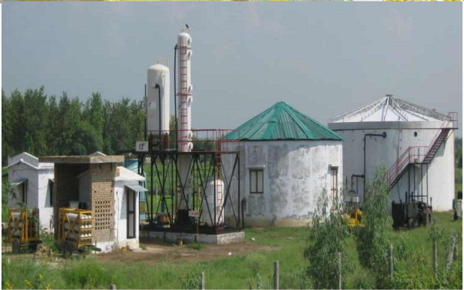
Biogas bottling project at Anand Energy, Vill. - Kallatiba, Dist.- Ferozepur (Punjab)
