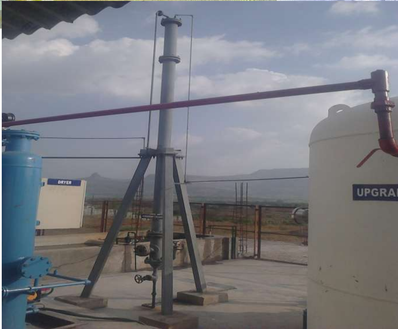
Biogas purification system (Water Scrubbing) at Talwade, Nasik
