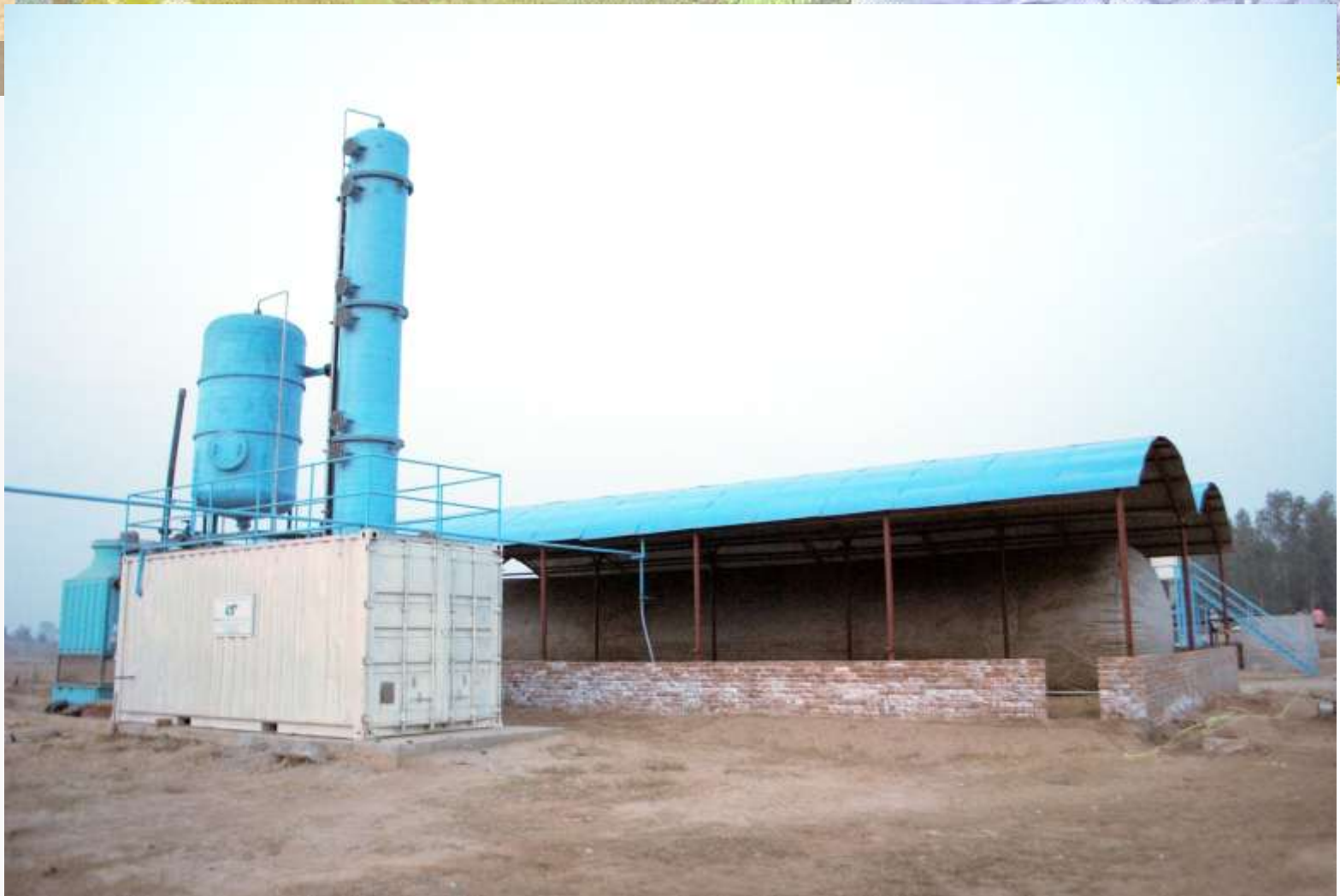
Biogas purification and storage system at Sask Energy, Village-Najabt Kukarian, P.O.-Lubaniawali, Tehsil & Dist. – Muktsar (Punjab)
