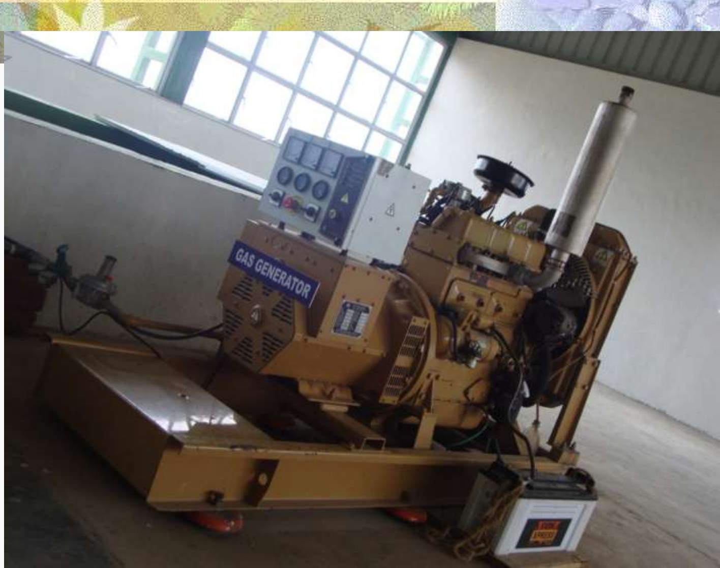
Biogas Genset at Talwade, Nasik
