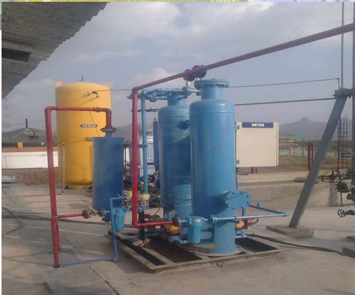
Biogas drier system at Talwade, Nasik
