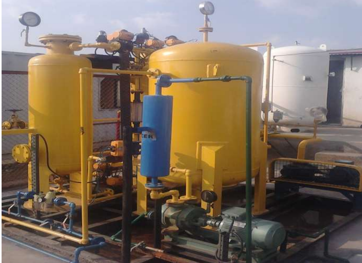
Biogas purification system (PSA Technology) at Talwade, Nasik
