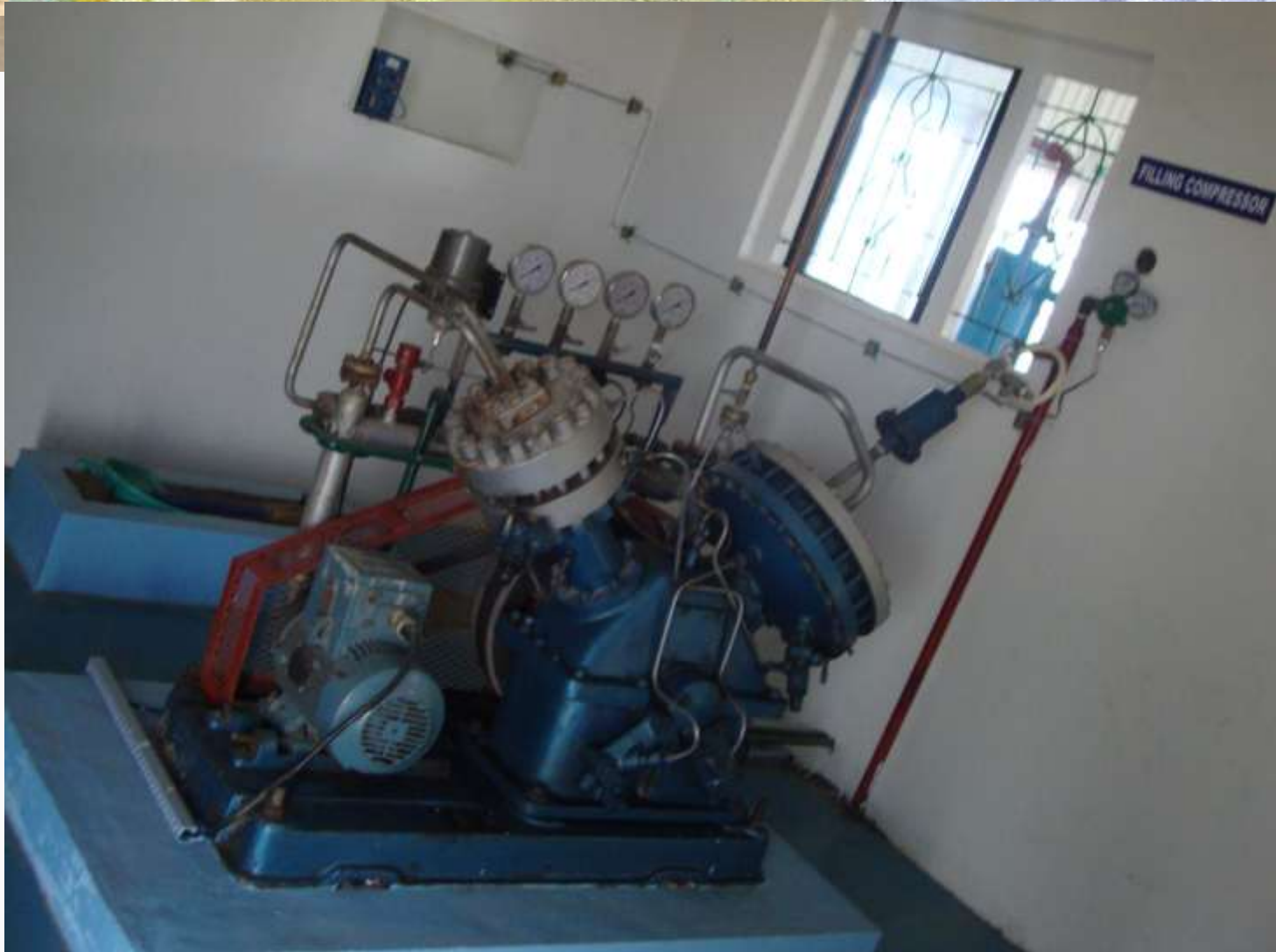
Biogas compressor at Talwade, Nasik
