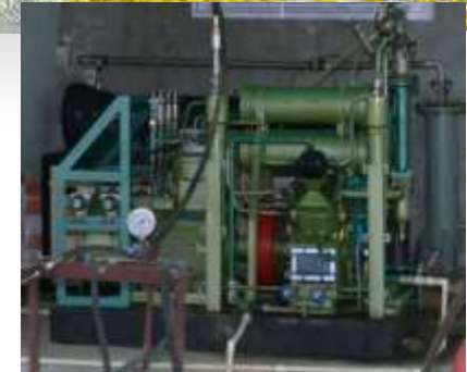
Biogas Bottling System
