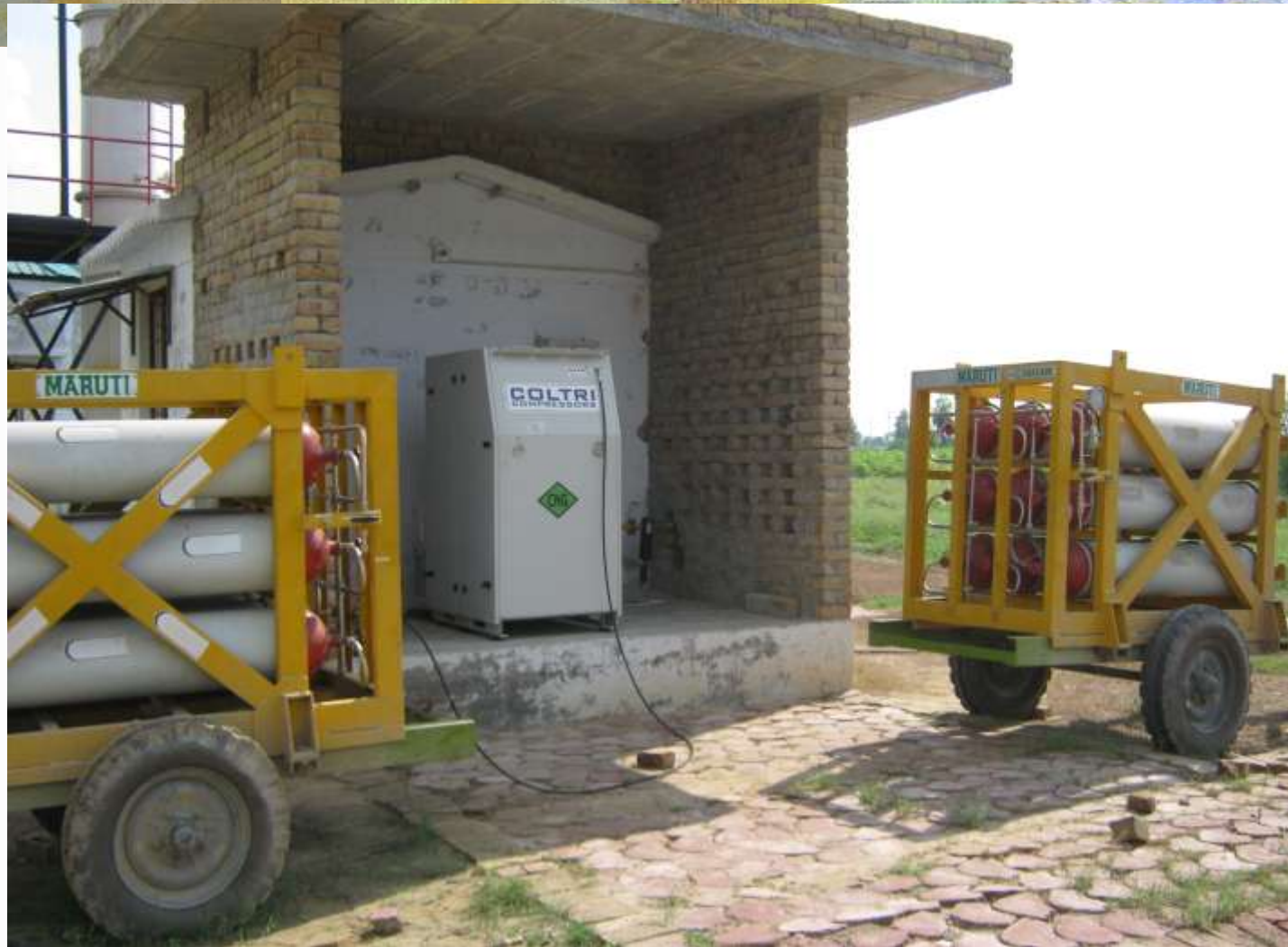
Cylinder cascade and compressor unit at Anand Energy, Vill. - Kallatiba, Dist.- Ferozepur (Punjab)
