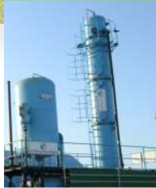
Biogas Purification system
