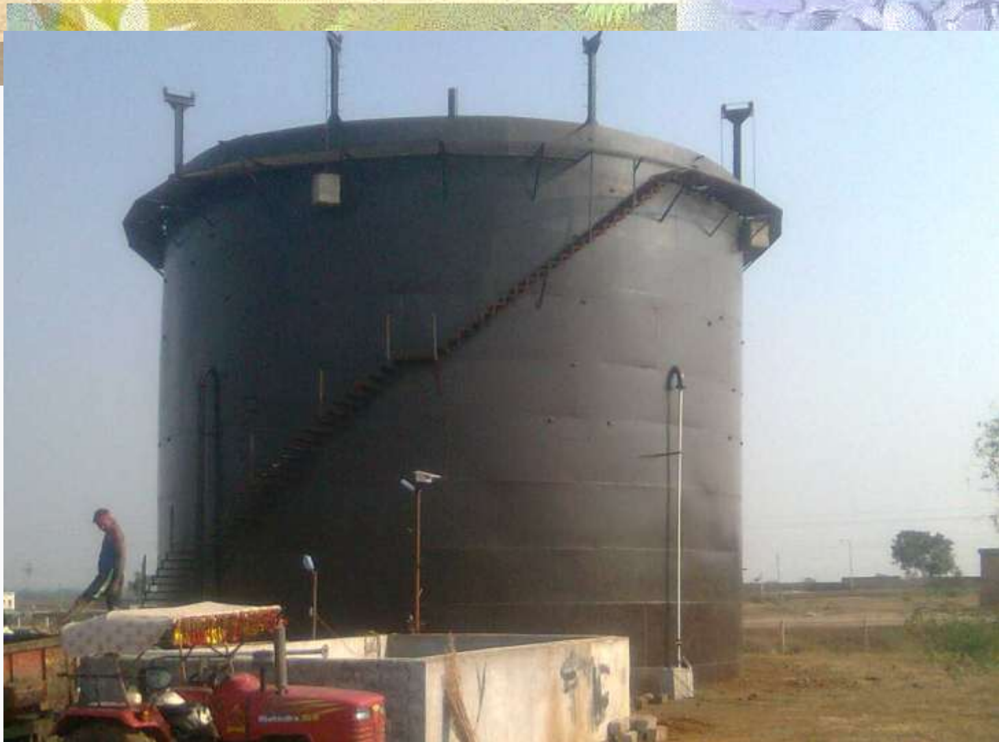
Biogas bottling project at R.G. Organics, Industrial Area Birkoni, Tehsil & Dist.- Mahasamund (Chhattisgarh) - under trial run
