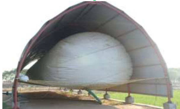
Biogas storage (Balloon)
