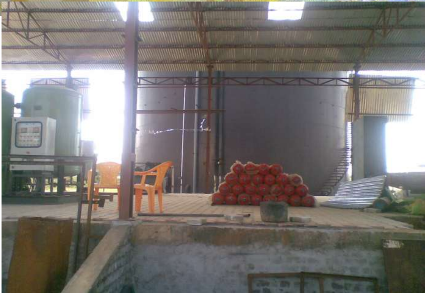
Biogas bottling project at R.G. Organics, Industrial Area Birkoni, Tehsil & Dist.- Mahasamund (Chhatisgarh) - under trial run
