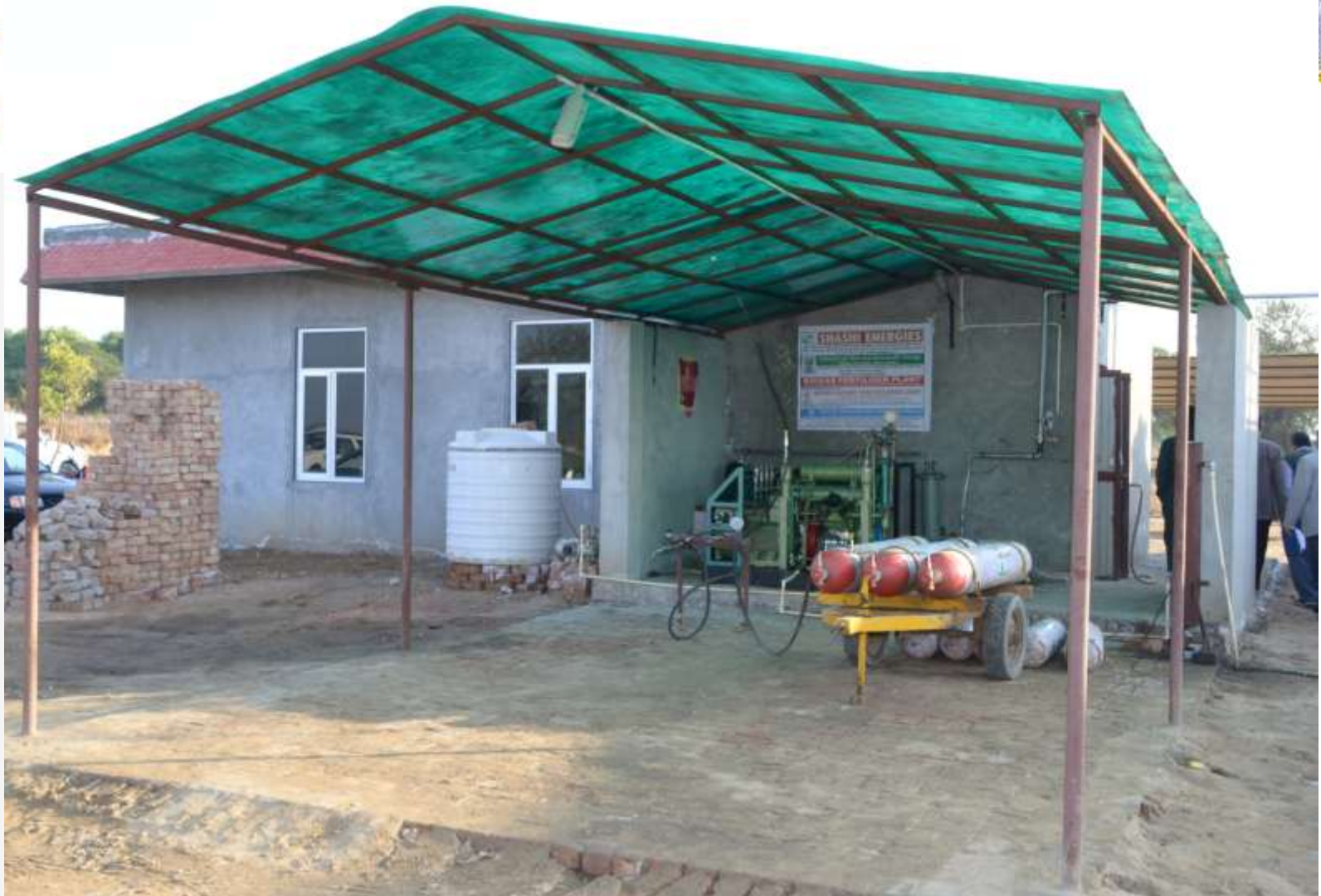
Biogas filling unit at Shashi Energies, Vill.-Tohana, near Green Valley Public School, Ratiya Road, Tehsil.-Tohana, Dist.-Fatehabad (Haryana)
