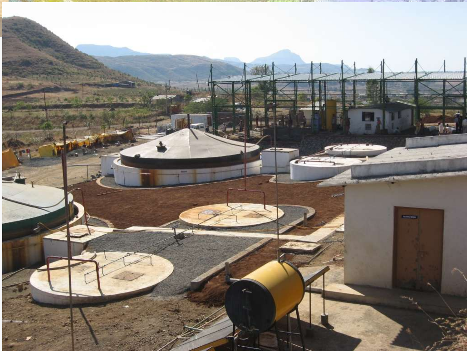
Biogas bottling project at Ashoka Biogreen Pvt. Ltd., Vill. - Talwade, Dist.-Nasik (Maharashtra)
