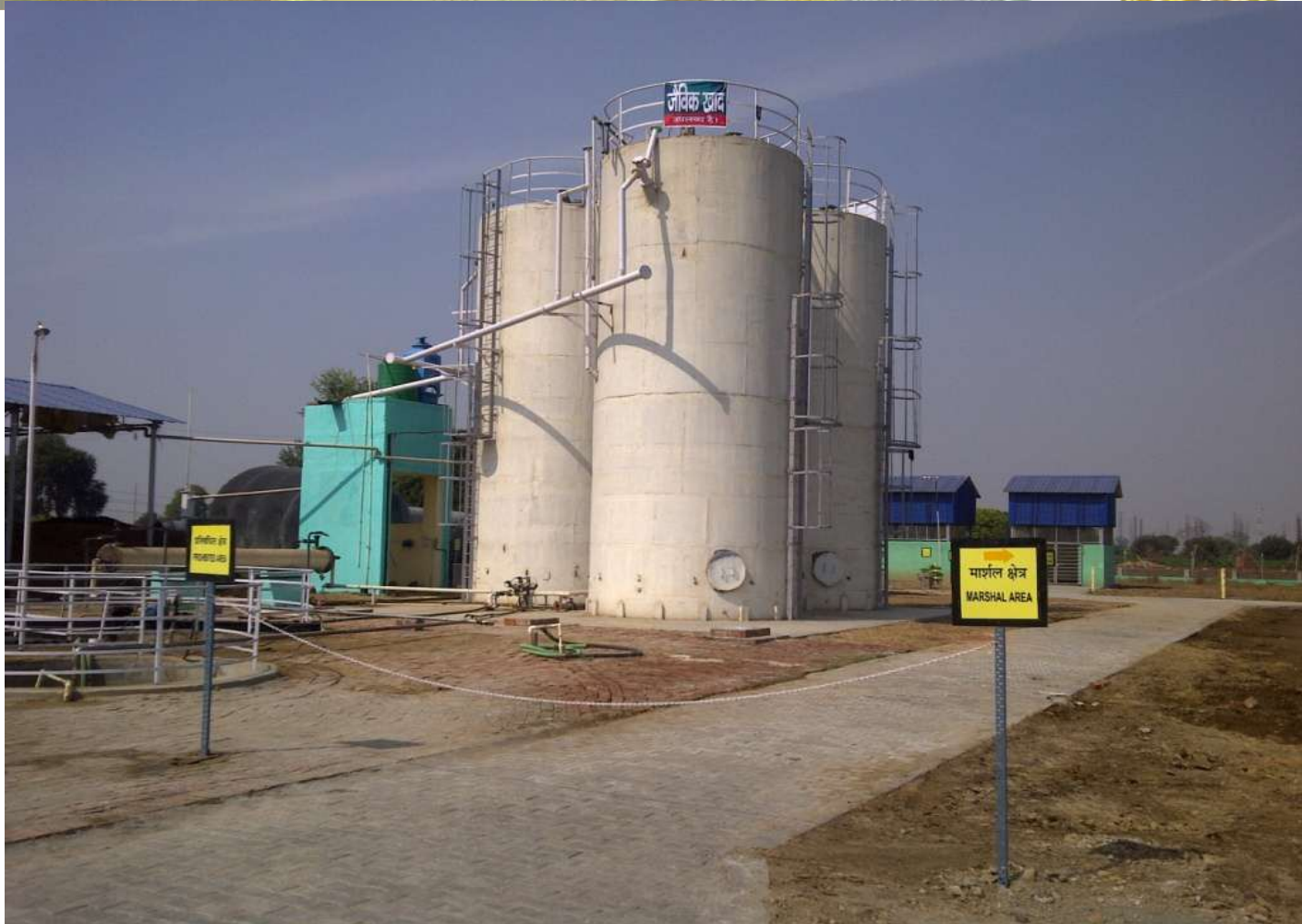
Biogas bottling project at Option Energy, Shree Haryana Gaushala, Vill./block – Hansi, Dist. Hissar (Haryana)
