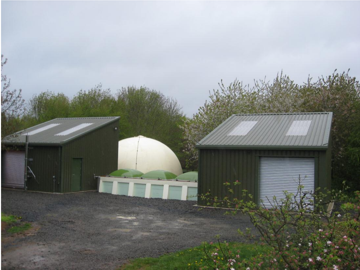
300 tonne per year community AD plant
