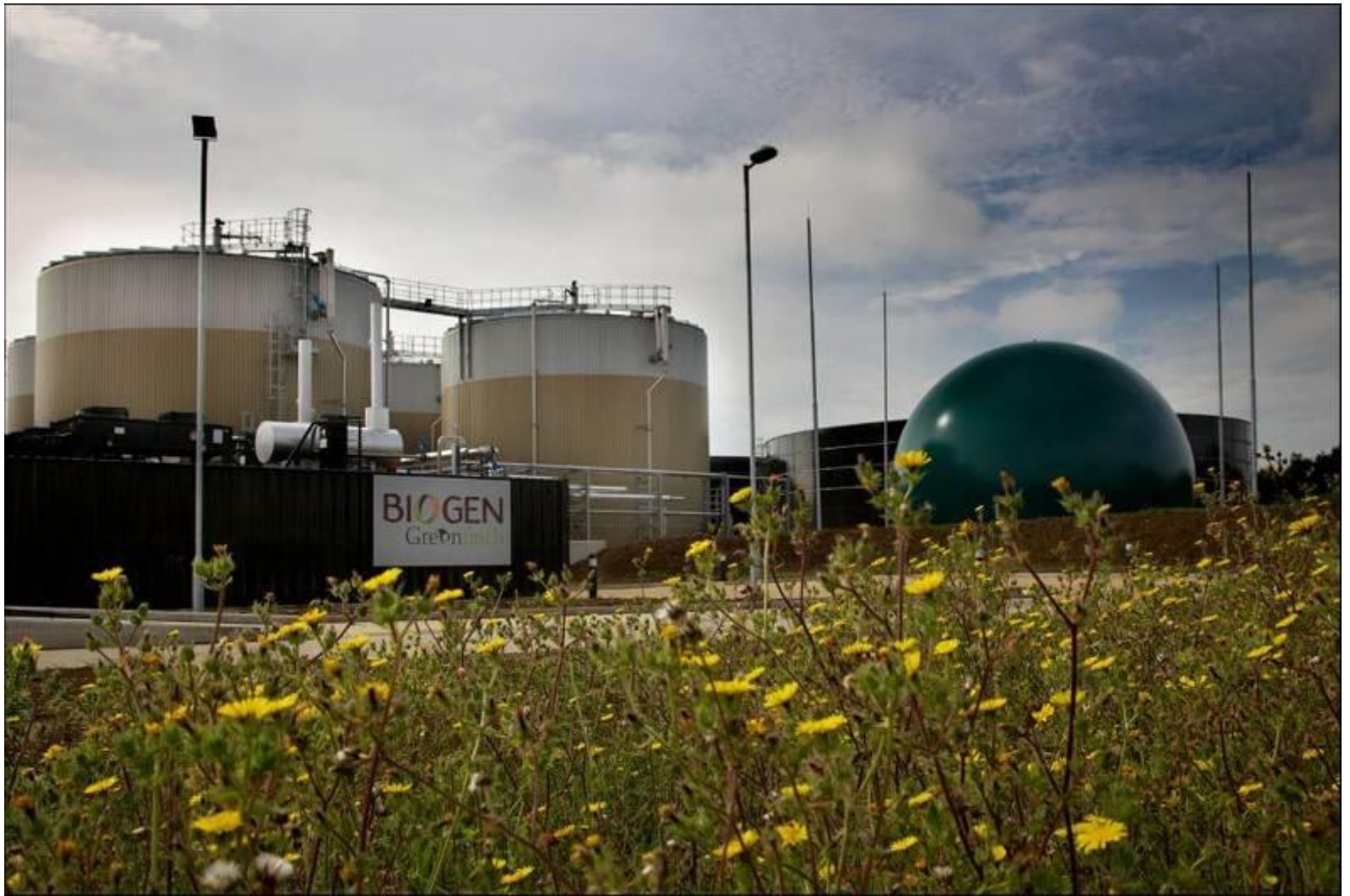
45,000 tonnes per year food waste AD plant in Northamptonshire
