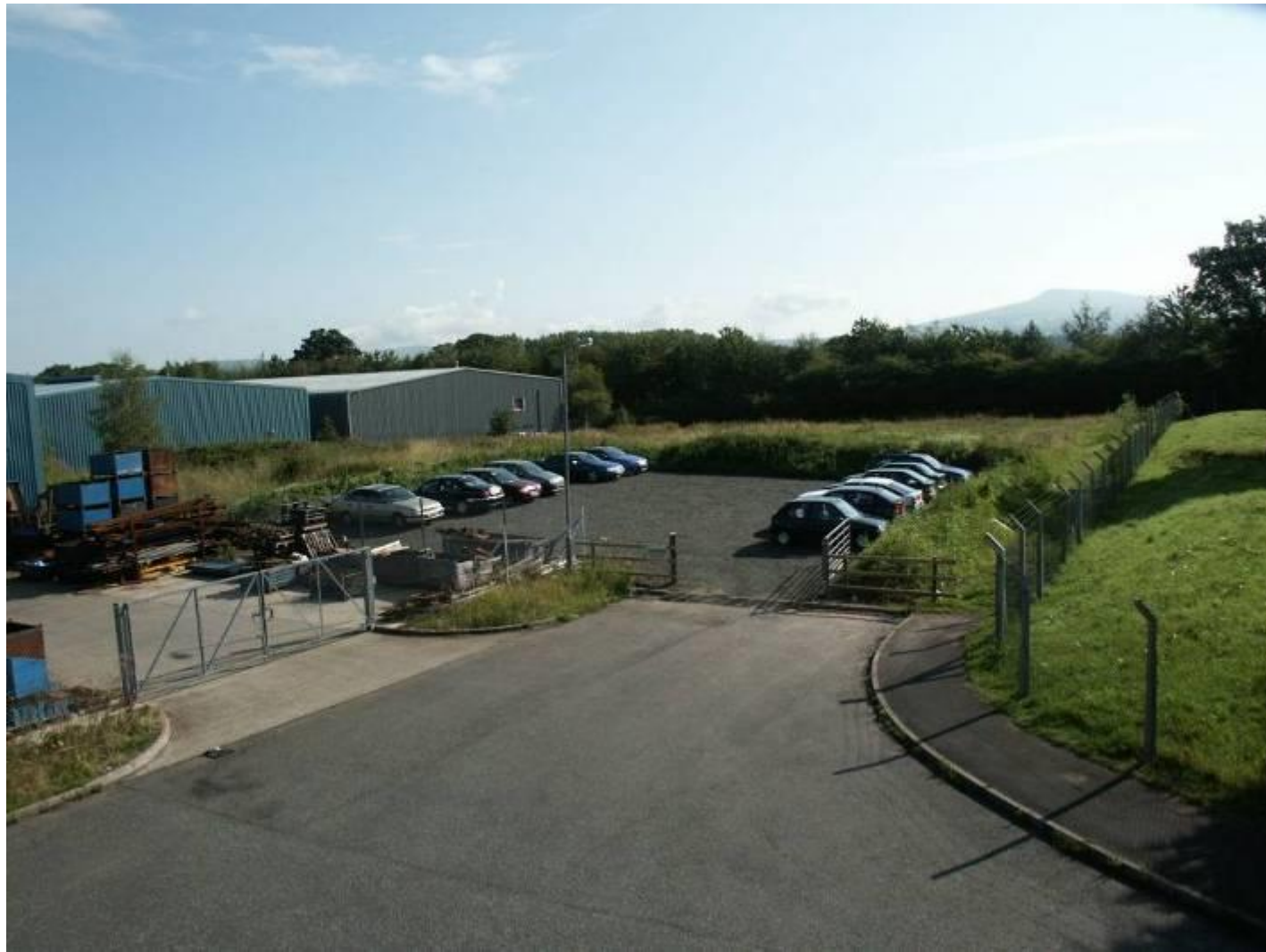
Ludlow biodigester site before construction
