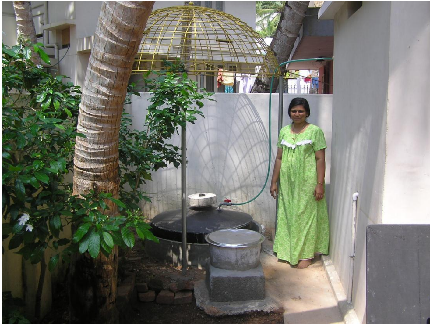
Household biogas plant in India
