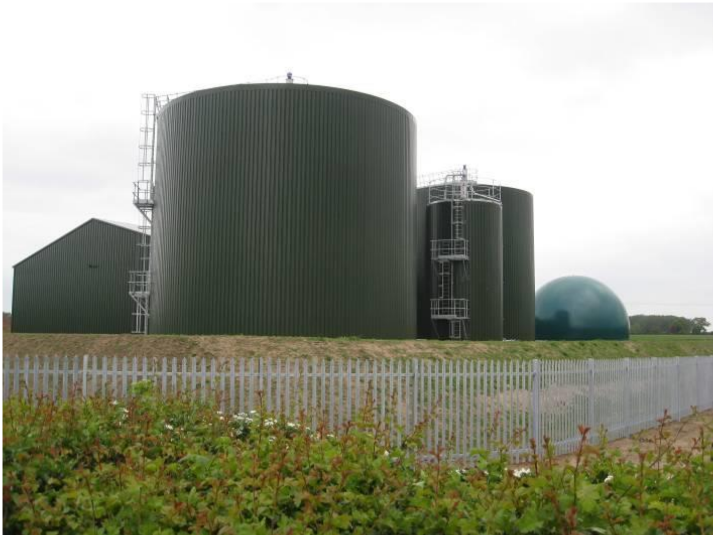
Co-digestion of food waste with cattle & pig manure in Shropshire
