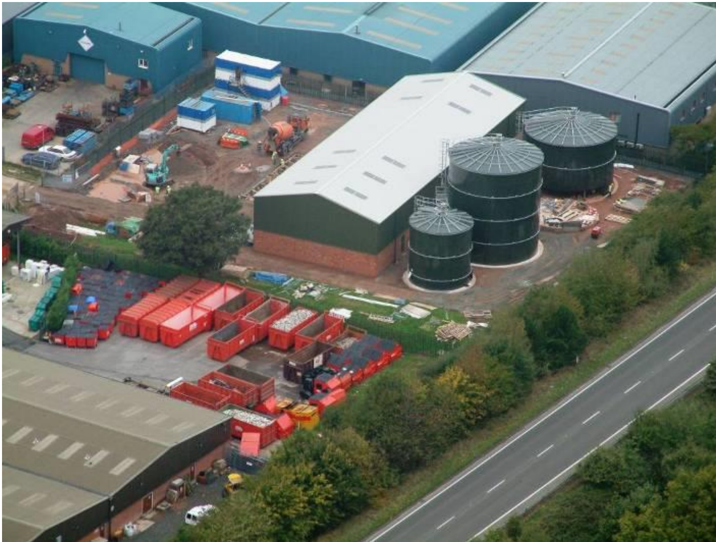
Ludlow biodigester under construction
