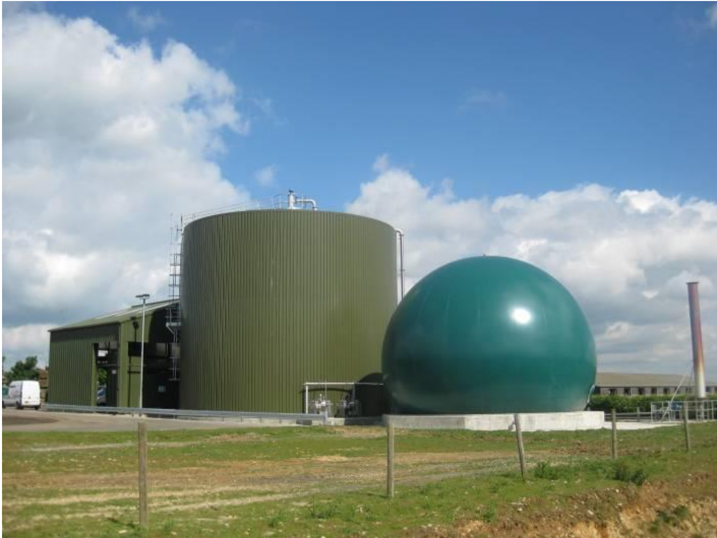
10,000 tonnes per year potato digester in Lincolnshire
